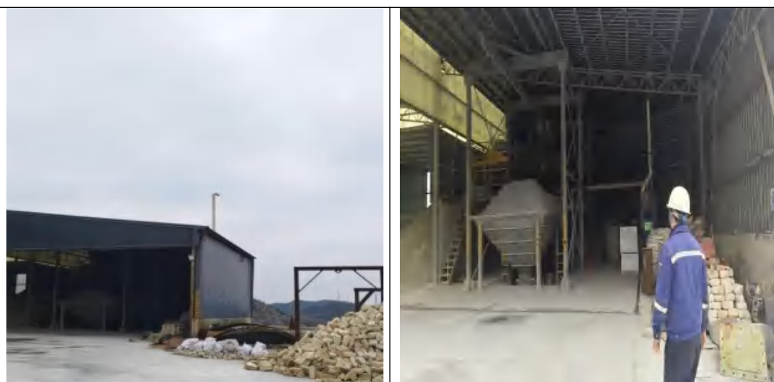
粗破车间废气排气筒
